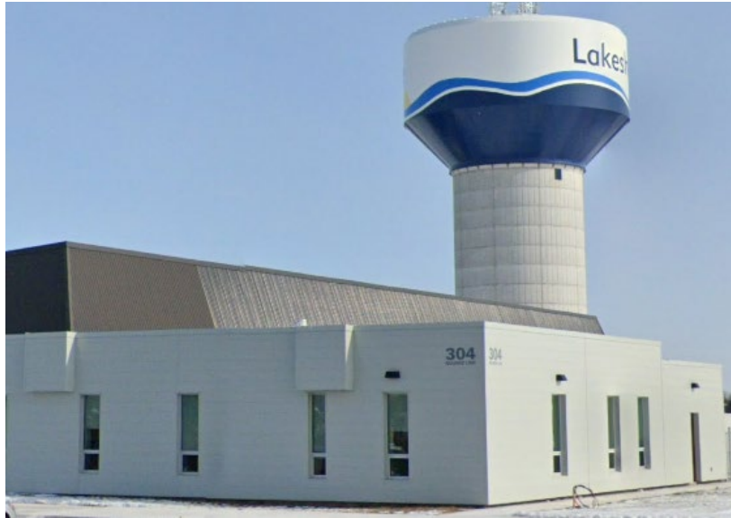
Operations Center (FMO), Rourke Line
