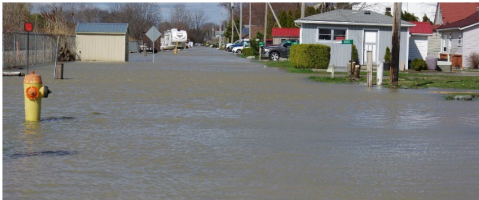
Caille Avenue after shoreline flooding occurred in September 2021
