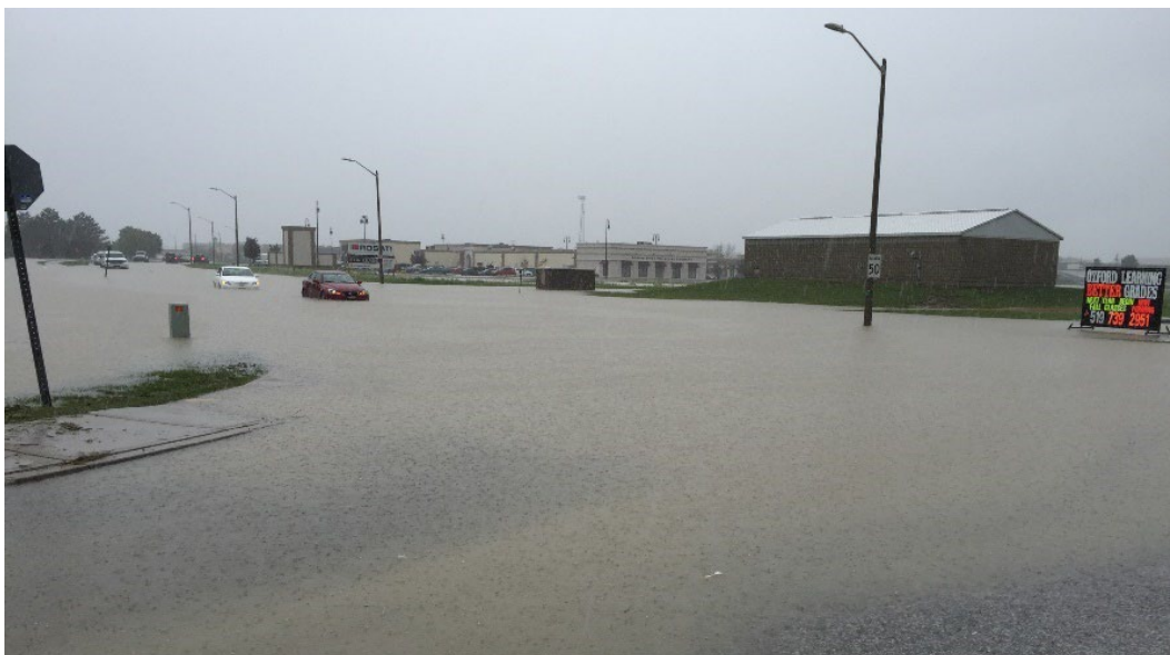
Patillo Road when flooding occurred on September 29, 2016
