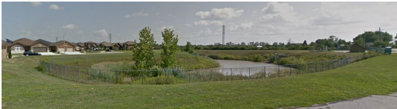
River Ridge Stormwater Management Pond
