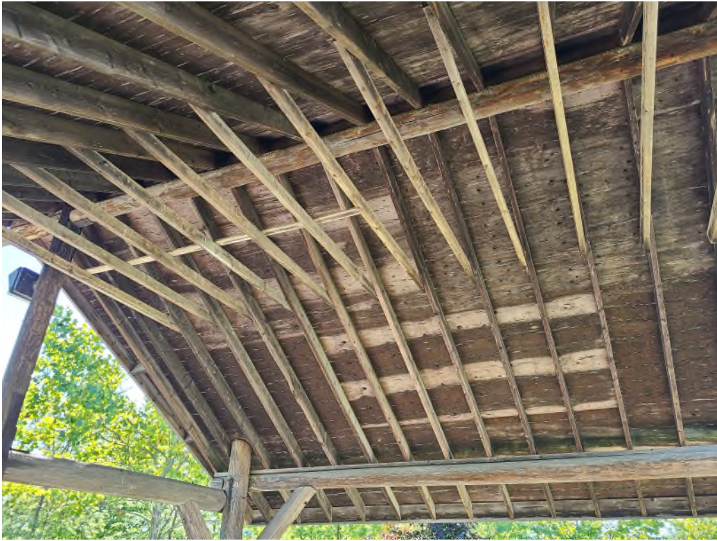
Photo #6: General View – Typical Roof Framing
