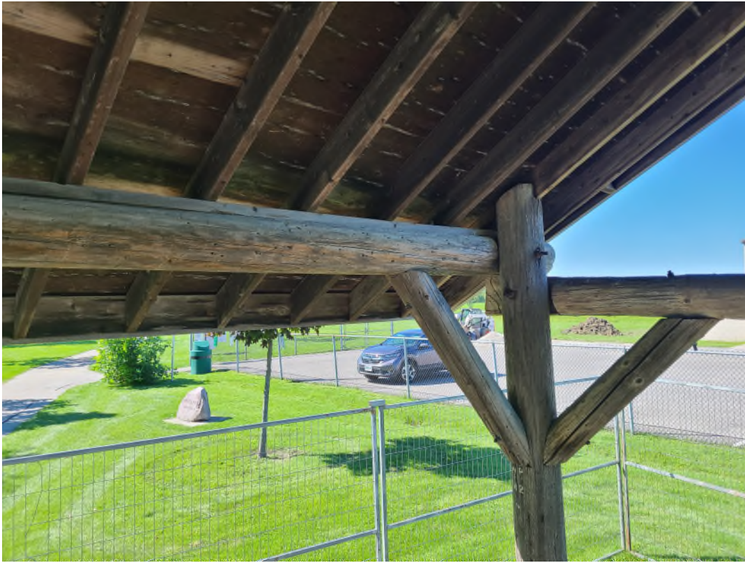
Photo #4: Typical Top-of-Post Connection
