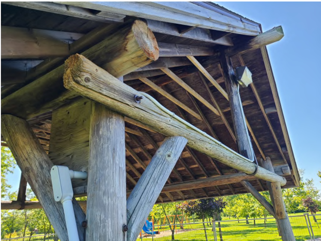
Photo #5: General View – Gazebo Framing along South Face
