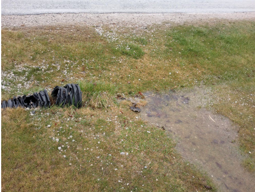
Figure 3: Picture showing subject property's drainage system split into a covered plastic culvert.
