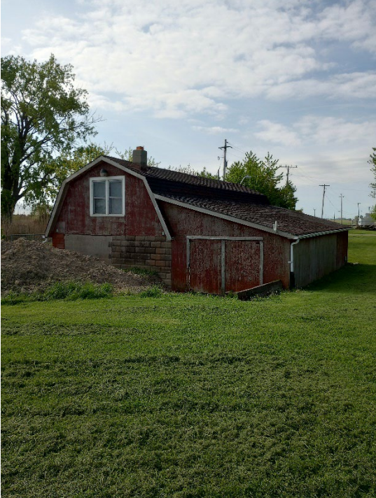
Figure 3: Rear view of existing building facing southeast.
