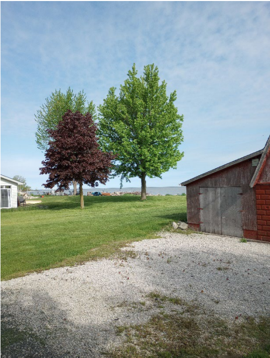
Figure 2: Northwest-facing view of existing building and property.
