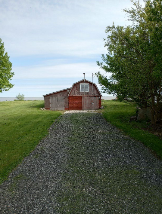
Figure 1: North-facing view of existing building from street.
