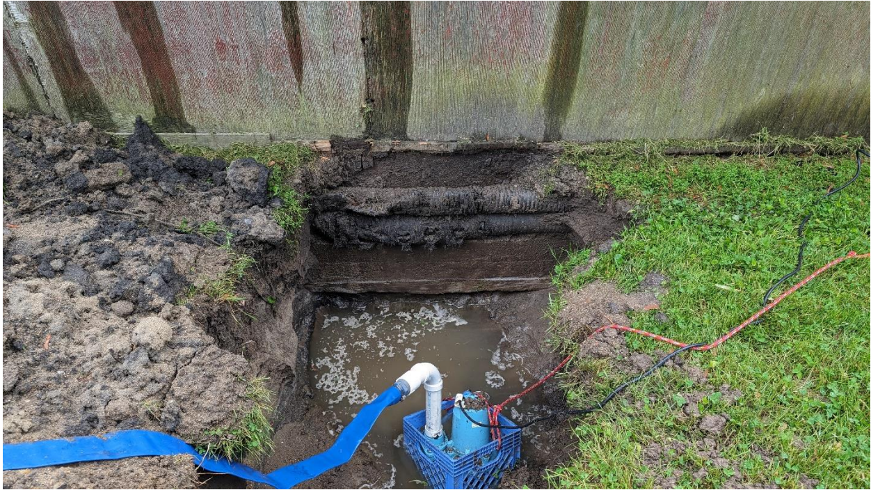
Figure 3 – Exposed footing on the West wall of the lean-to portion.
