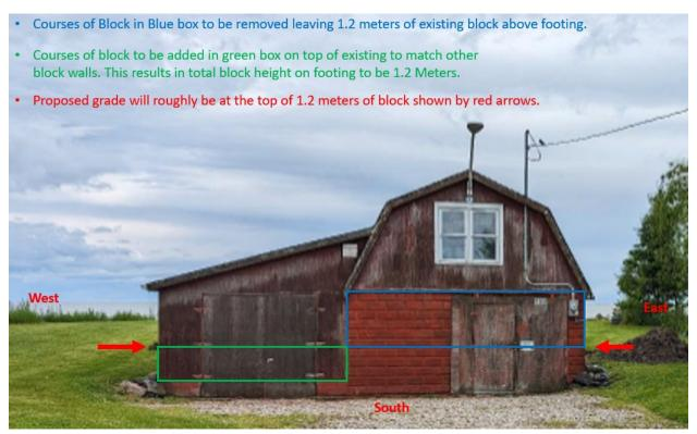
This follows the structural report as it states - "The number of block units added to the existing lean- to block masonry foundation wall should be limited to the minimum number of blocks required to reach above the proposed grade – approximately 1.2 metres."
