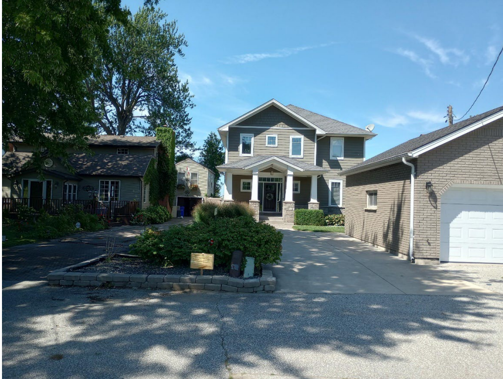
Figure 3: Subject property and neighbouring property to the west as seen from street, facing north.
