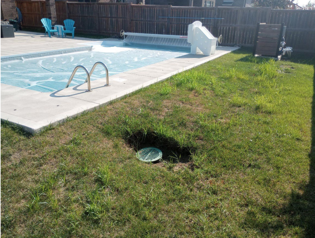
Figure 3: Existing drain in rear yard, located between pool and rear lot line.
