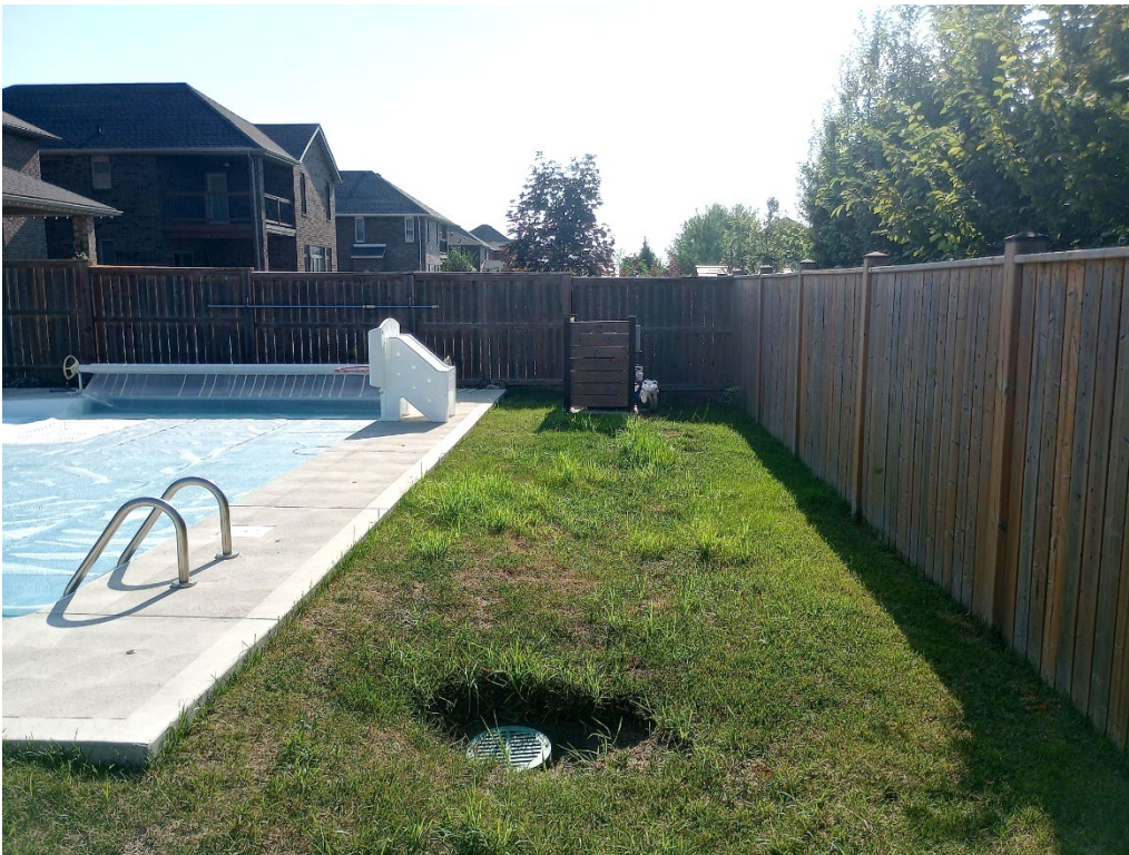
Figure 4: East-facing view of existing drain, pool, and pool equipment in southern portion of rear yard.
