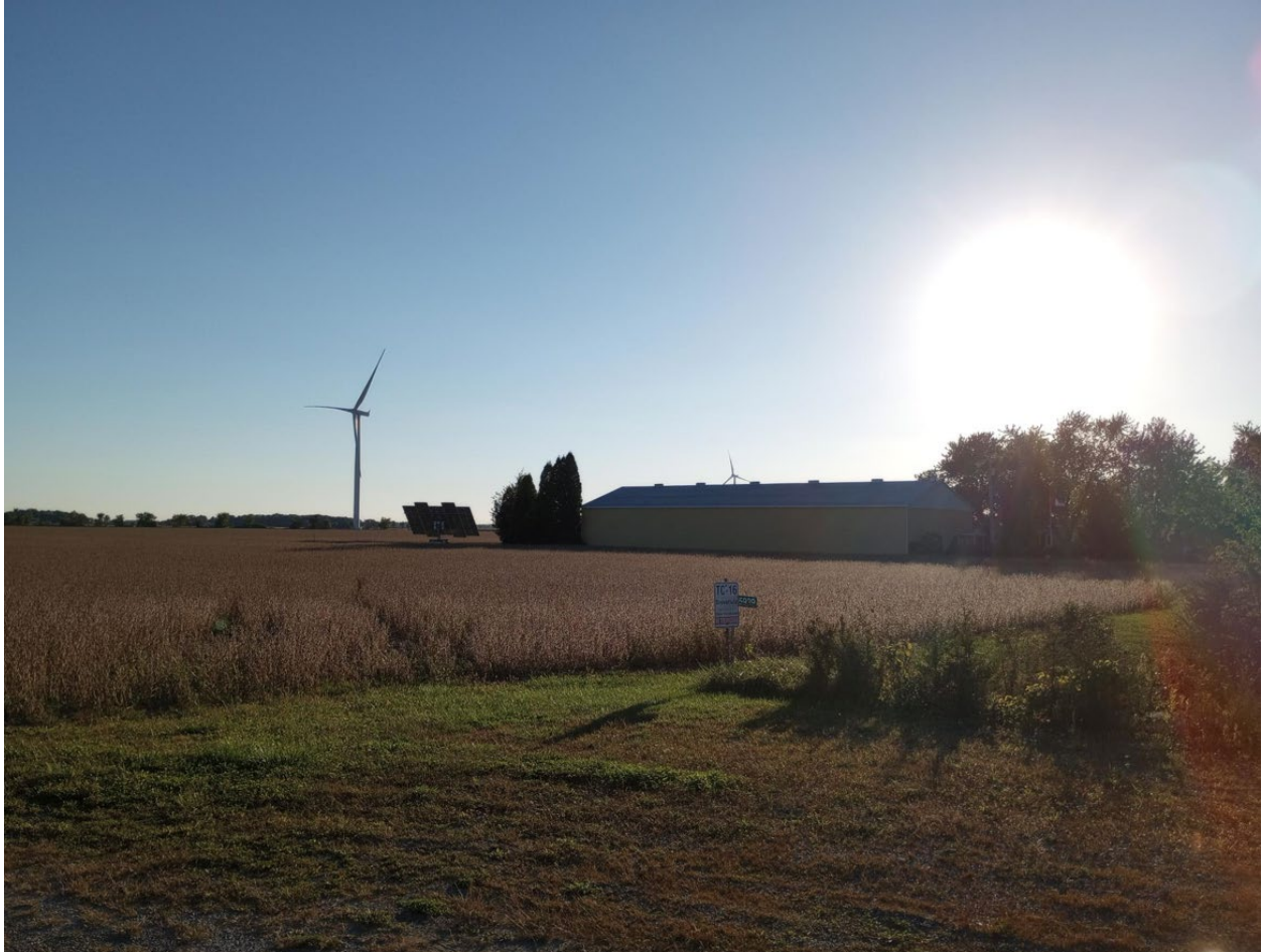
Picture of one of the buildings on the subject property looking southwest from the northeast corner of the property
