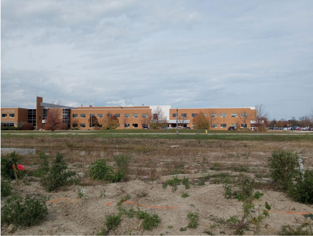
Picture of the school located northwest of the semi-detached dwellings under construction
