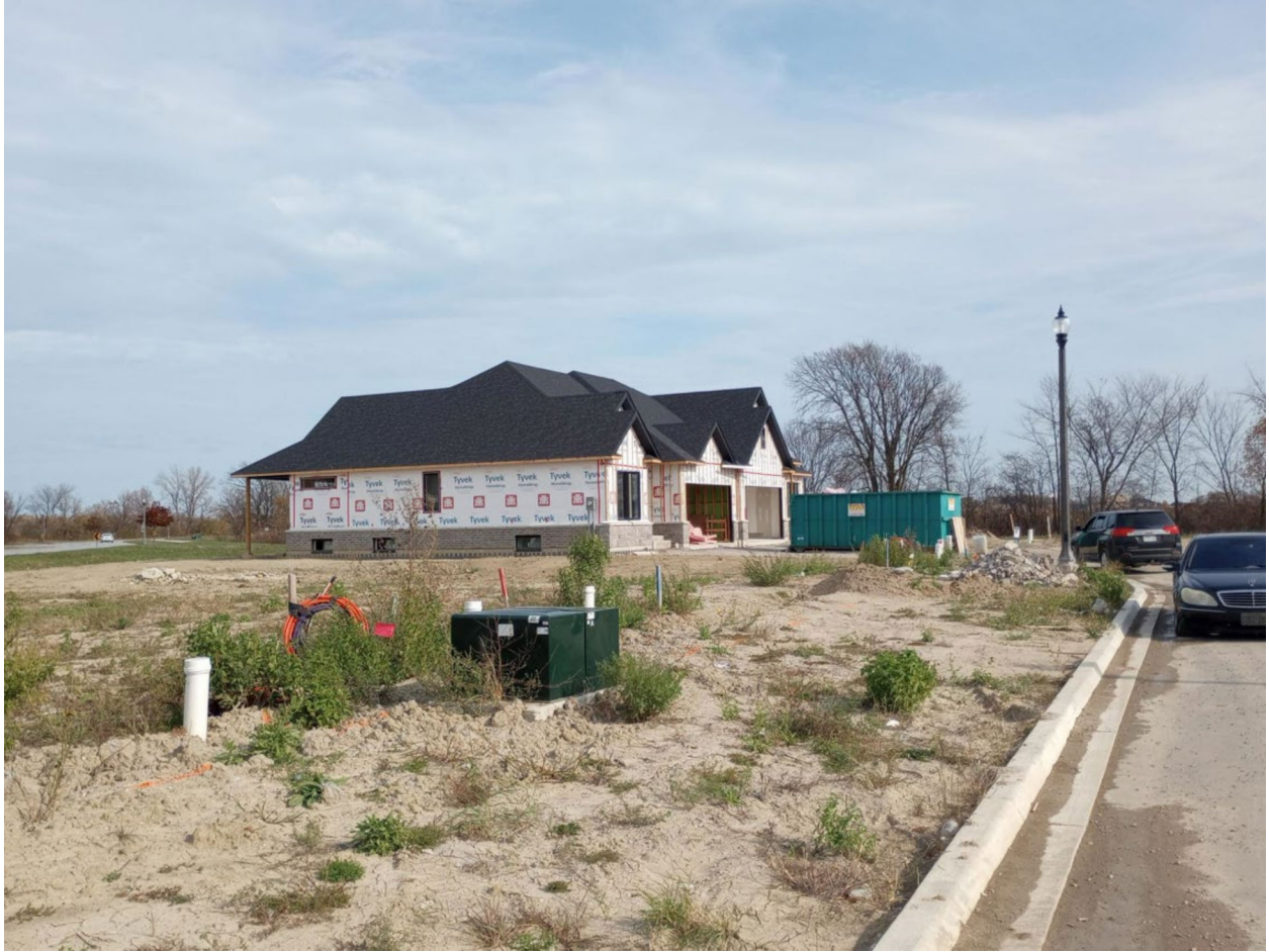
Picture of the semi-detached dwellings under development looking east
