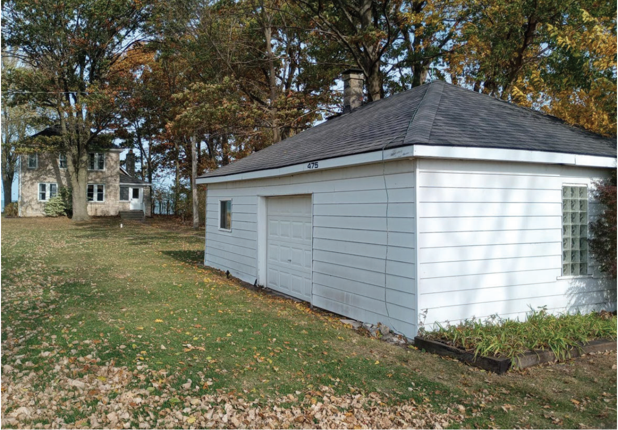
Picture of existing buildings on 475 Charron Beach Road looking north
