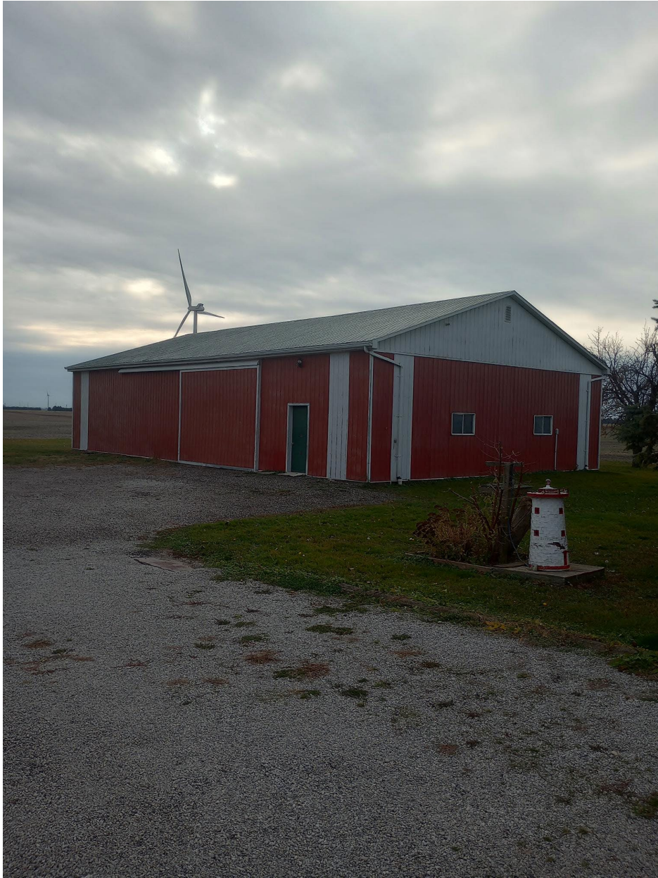
Looking southwest towards the accessory structure located near the southwest corner of the proposed severed lot
