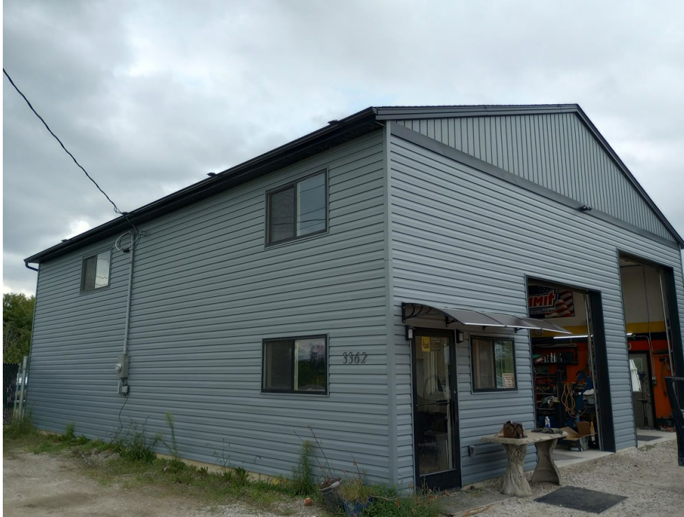
Picture of the accessory building looking northeast from the driveway
