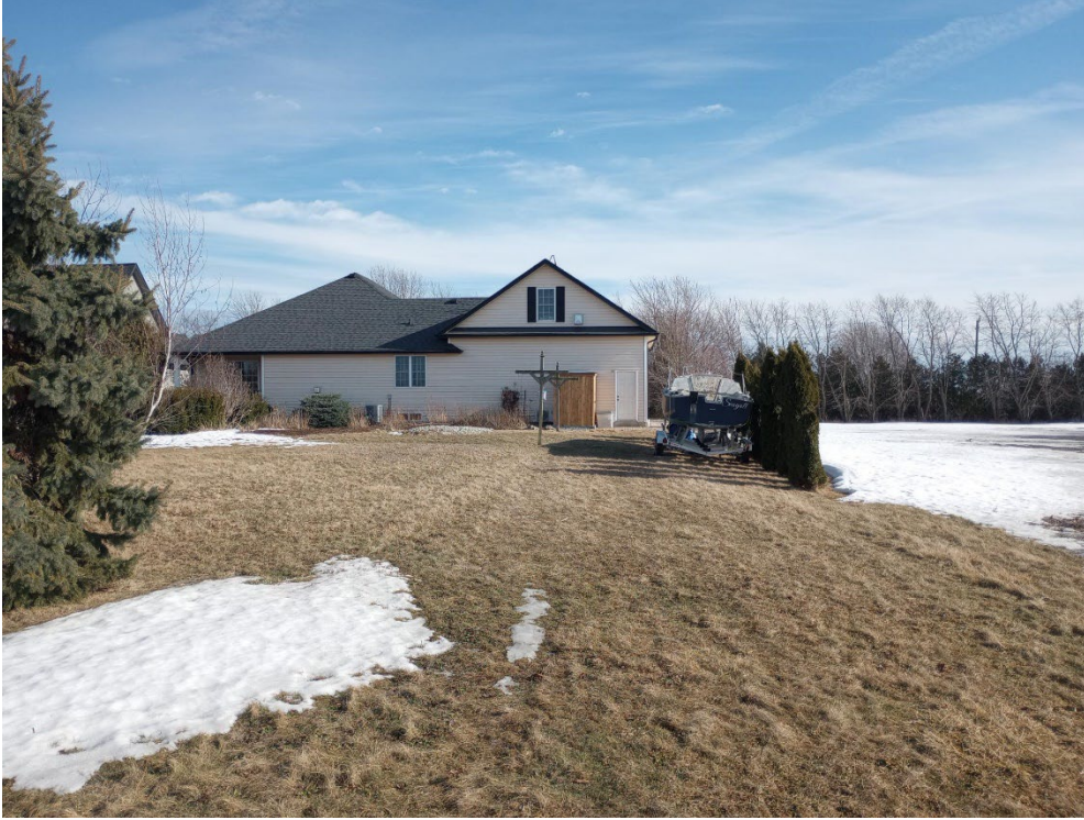
Looking towards the existing house from the proposed accessory building location.
