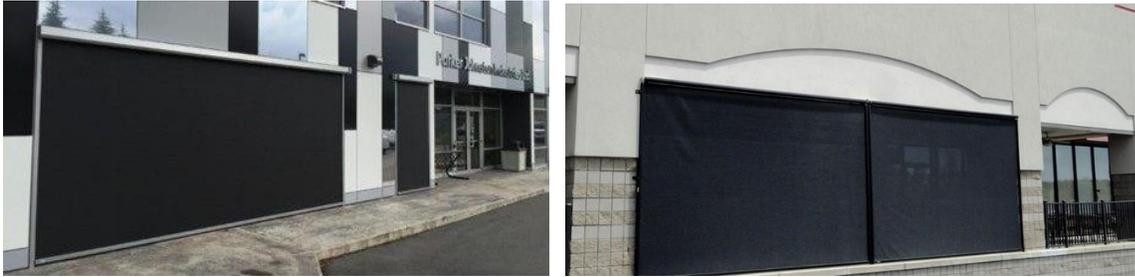
Installing retractable screens would eliminate the heat from the East facing windows during the hot summer months. These manually operated retractable screens would be down, covering the windows in the hot summer months, and cleaned/retracted back up under the soffits in the fall, winter months.
