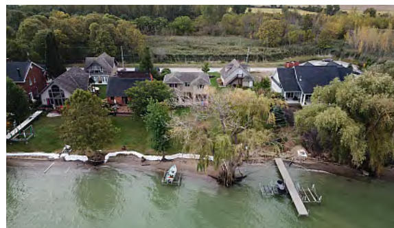
Beach Shoreline with Sand Bags
