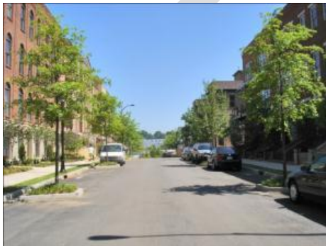
Figure 26: Image from Wallace Woods Concept Plan Report – Sample Urban Residential Local Road
