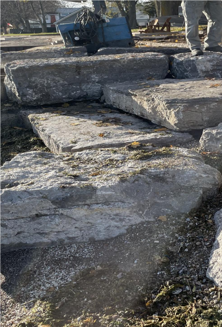
Stepped armour stone to allow for access
