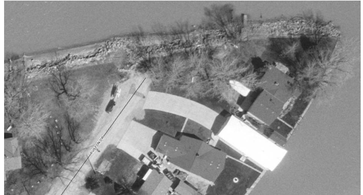
Ruston Drive North Shoreline in 2004
