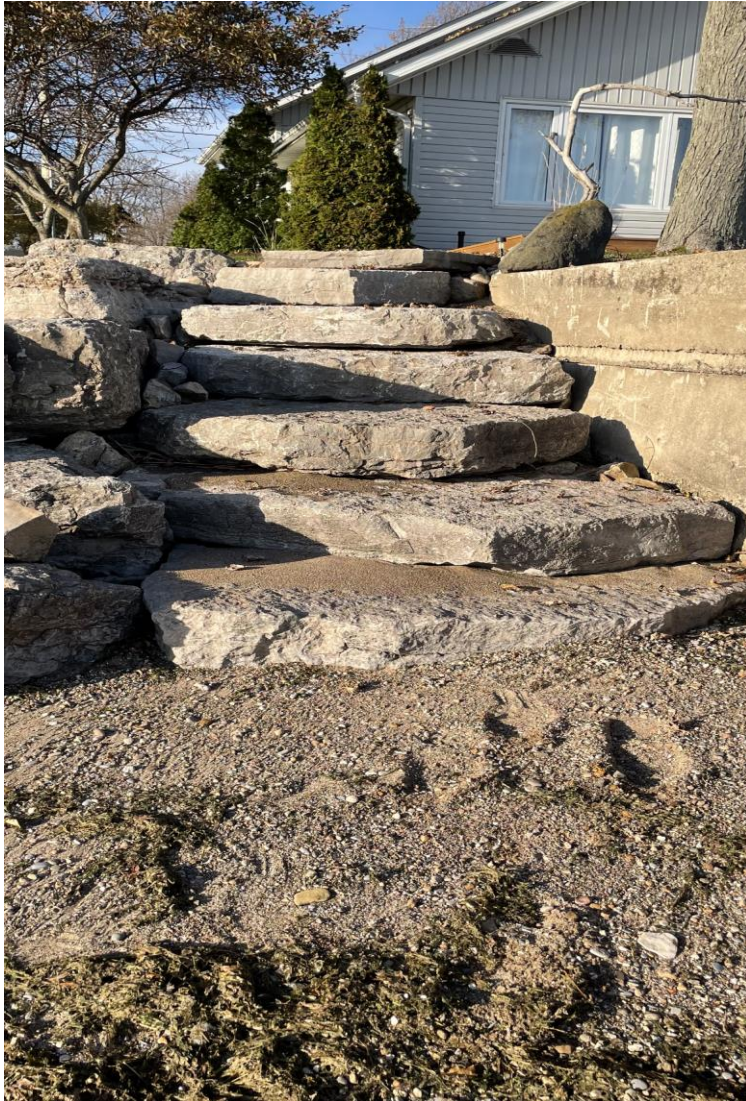
Stepped armour stone to allow for access
