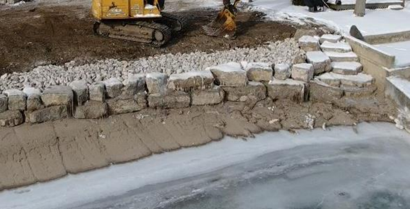
After Shoreline Protection & Access
