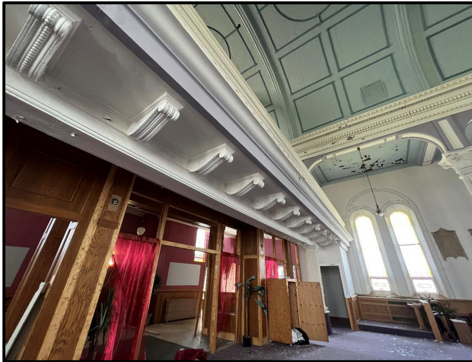
Image 34: 7119 Tecumseh Road Interior Detail – Balcony Bracketing (Photo taken July 22, 2022)
