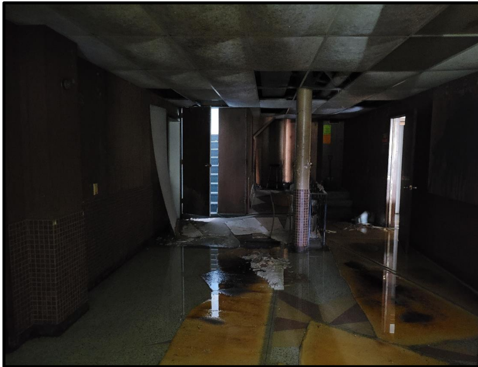
Image 46: 7119 Tecumseh Road Interior – Basement Hall (Photo taken July 22, 2022)
