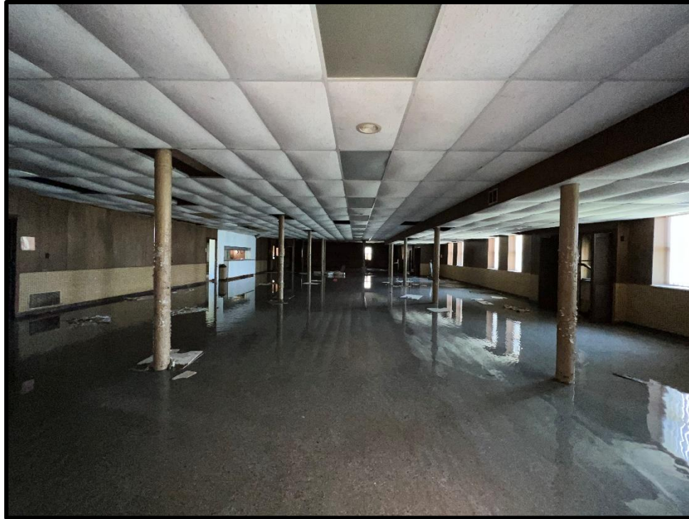
Image 47: 7119 Tecumseh Road Interior – Basement (Photo taken July 22, 2022)
