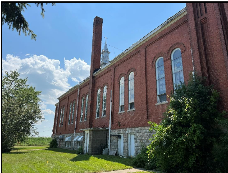
Image 14: 7119 Tecumseh Road Exterior – East Elevation (Photo taken July 22, 2022; Facing Southwest)
