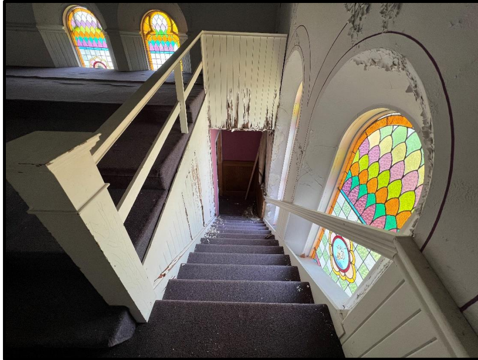
Image 37: 7119 Tecumseh Road Interior – East Stairs to Balcony (Photo taken July 22, 2022)
