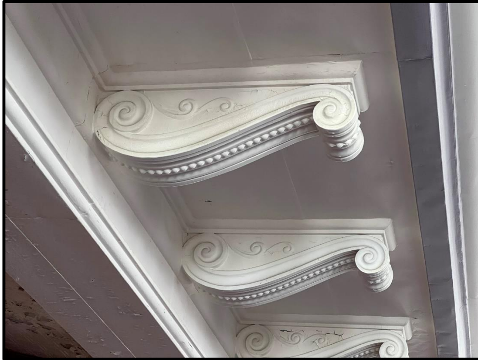
Image 35: 7119 Tecumseh Road Interior Detail – Pressed Tin Bracketing Under Balcony (Photo taken July 22, 2022)
