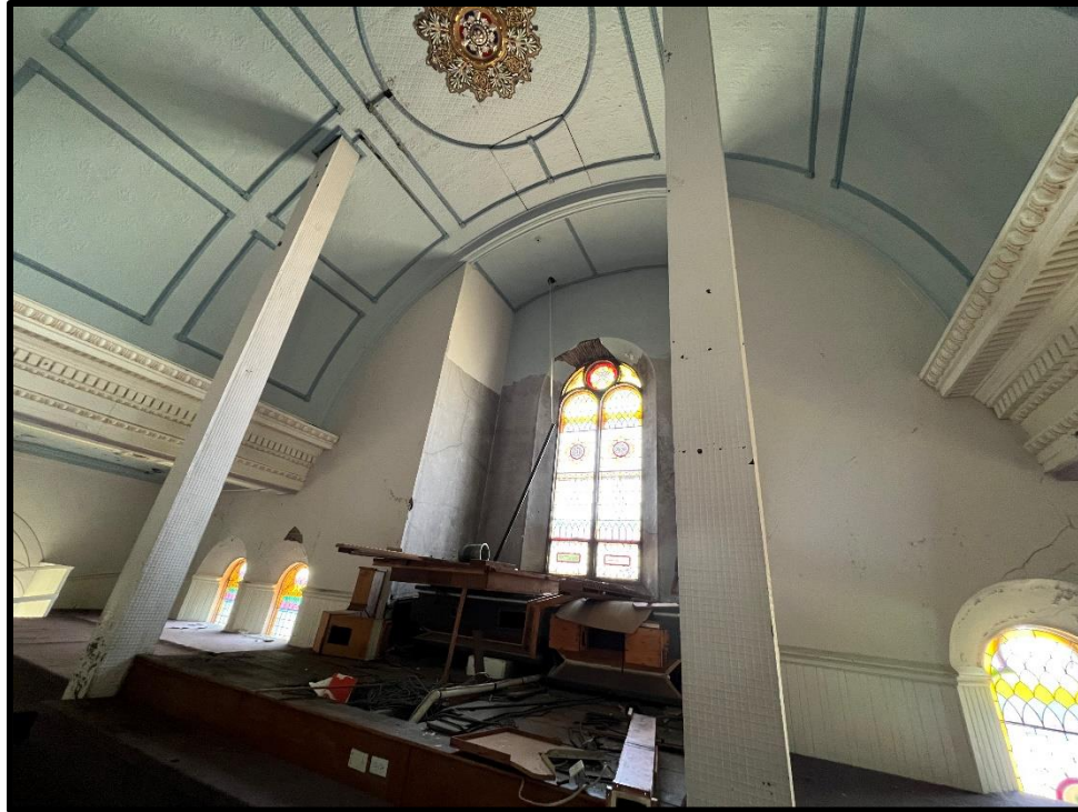
Image 41: 7119 Tecumseh Road Interior – Balcony (Photo taken July 22, 2022)
