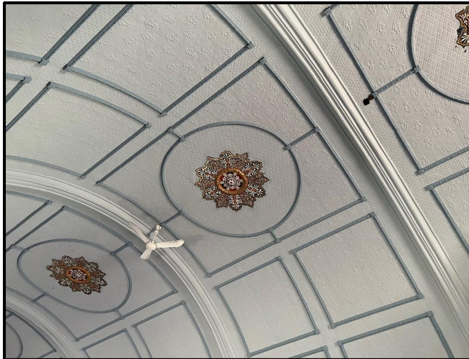
Image 28: 7119 Tecumseh Road Interior Detail – Pressed Tin Ceiling (Photo taken July 22, 2022)
