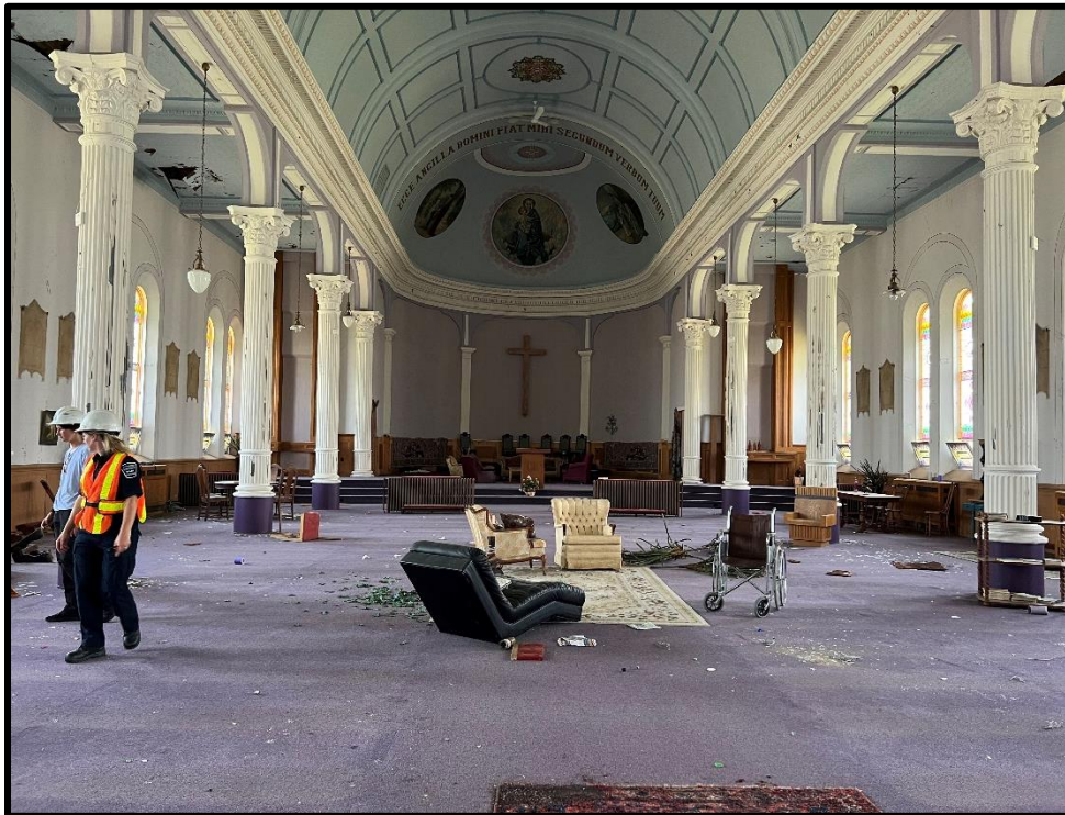
Image 22: 7119 Tecumseh Road Interior – Nave (Photo taken July 22, 2022)
