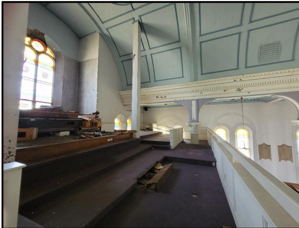
Image 40: 7119 Tecumseh Road Interior – Balcony (Photo taken July 22, 2022)
