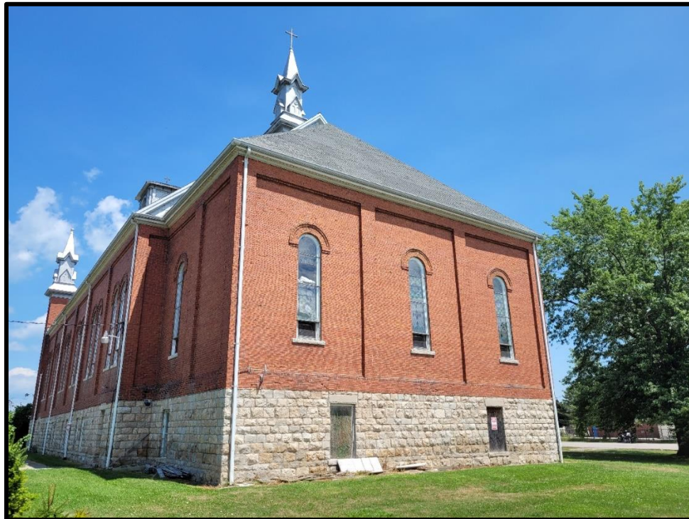
Image 16: 7119 Tecumseh Road Exterior – South (Rear) Elevation (Photo taken July 22, 2022; Facing Northeast)
