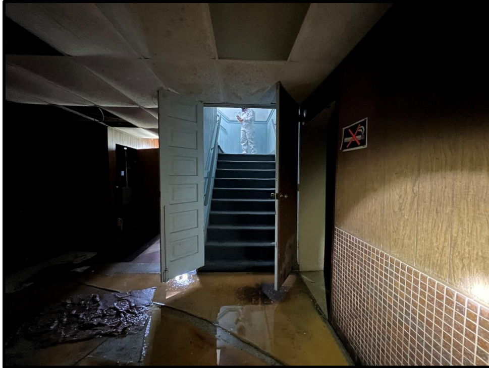
Image 45: 7119 Tecumseh Road Interior – Basement Hall (Photo taken July 22, 2022)
