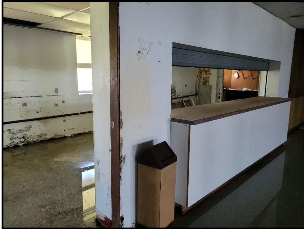
Image 51: 7119 Tecumseh Road Interior – Basement Kitchen (Photo taken July 22, 2022)
