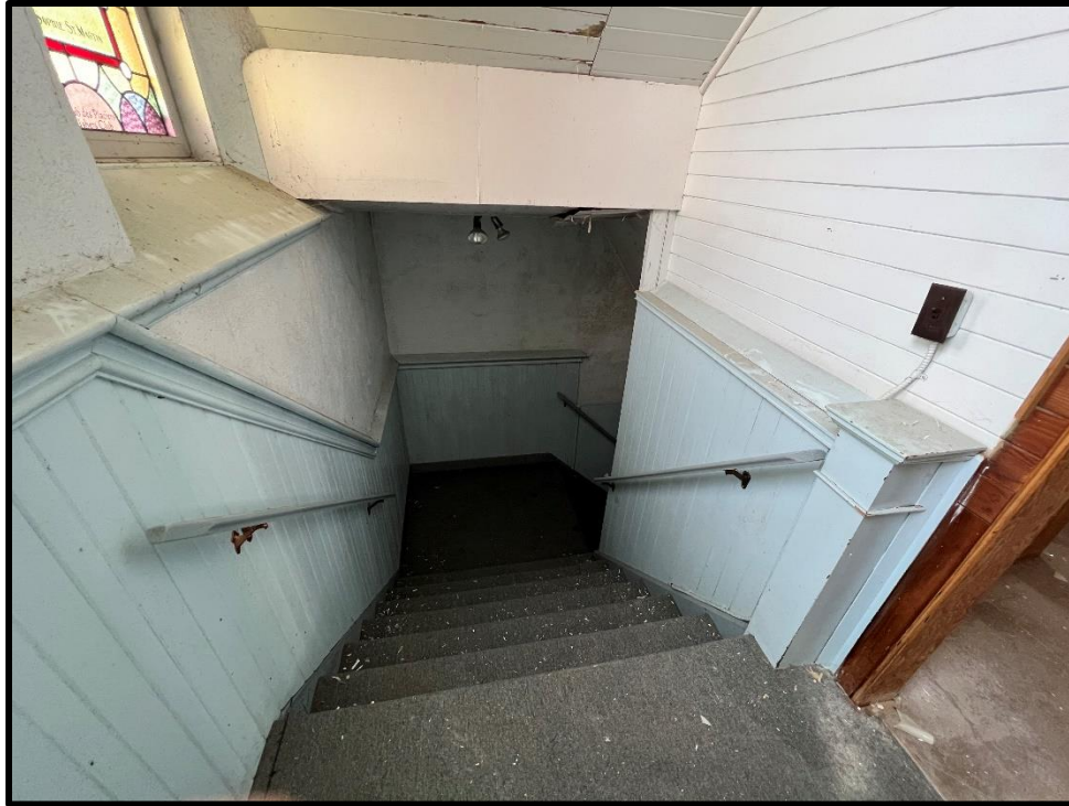
Image 43: 7119 Tecumseh Road Interior – Stairs to Basement (Photo taken July 22, 2022)
