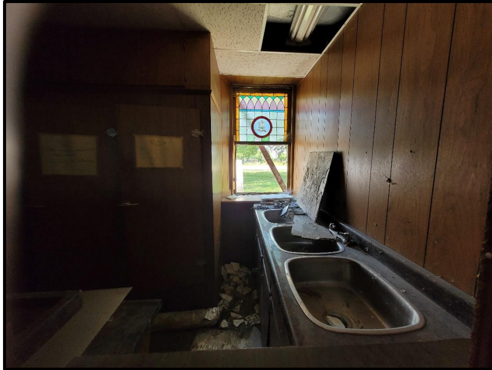
Image 53: 7119 Tecumseh Road Interior – Basement Kitchen (Photo taken July 22, 2022)
