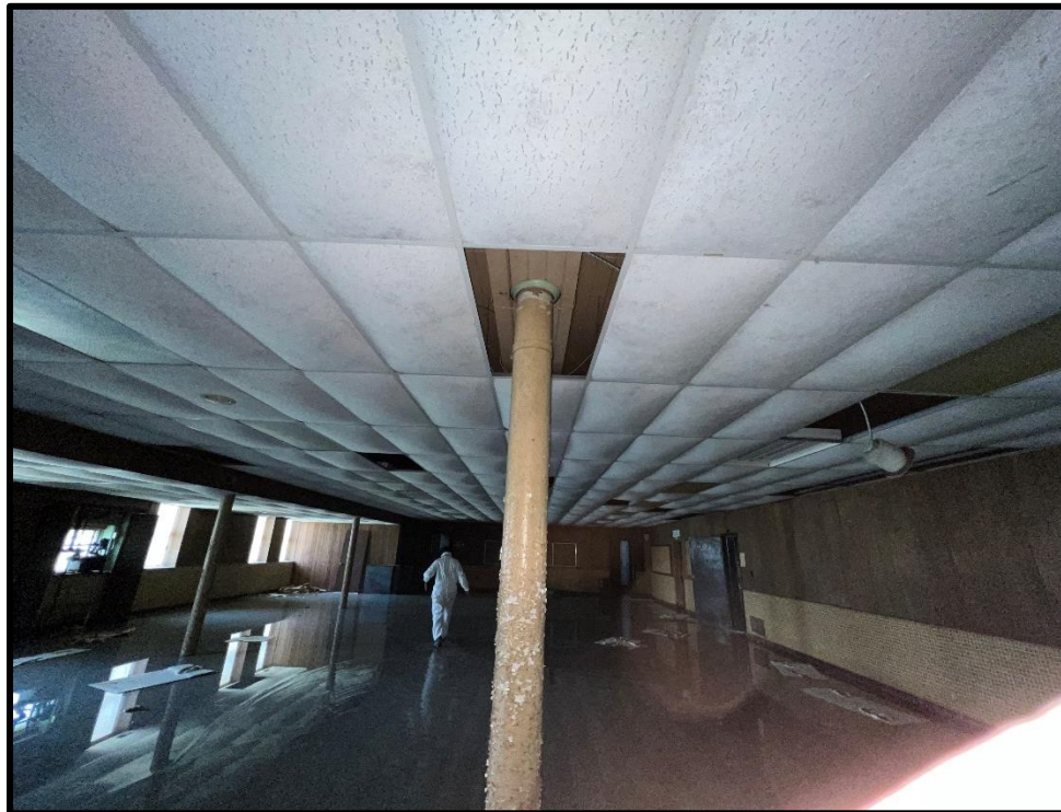
Image 48: 7119 Tecumseh Road Interior – Basement Columns (Photo taken July 22, 2022)
