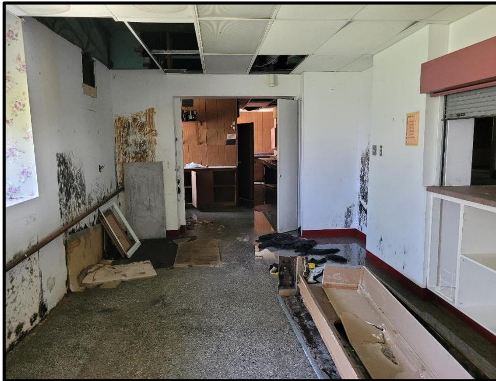
Image 52: 7119 Tecumseh Road Interior – Basement Kitchen (Photo taken July 22, 2022)
