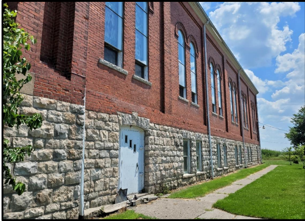
Image 17: 7119 Tecumseh Road Exterior – West Elevation (Photo taken July 22, 2022; Facing South)
