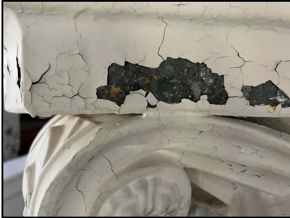
Image 39: 7119 Tecumseh Road Interior Detail – Former Gold Paint Finish on Columns (Photo taken July 22, 2022)
