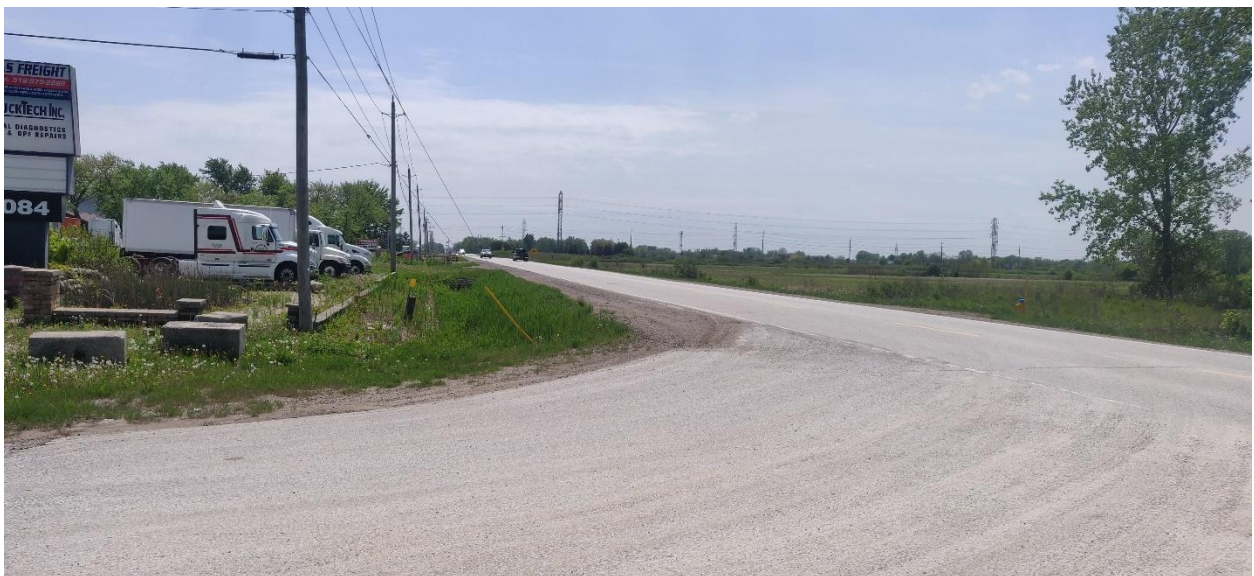
Figure 2 – Existing Site Driveway at 2084 Manning Road – Sight Line to the South
