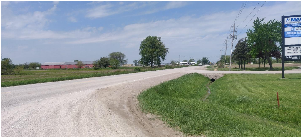
Figure 1 – Existing Site Driveway at 2084 Manning Road – Sight Line to the North
